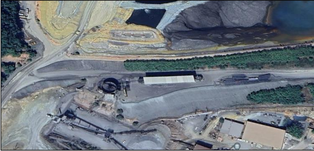
Figure 4 Aerial view of the Dominican Republic filtration plant
