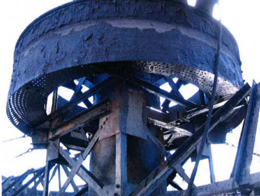
Figure 2: Original thickener feedwell (prior to upgrade)
