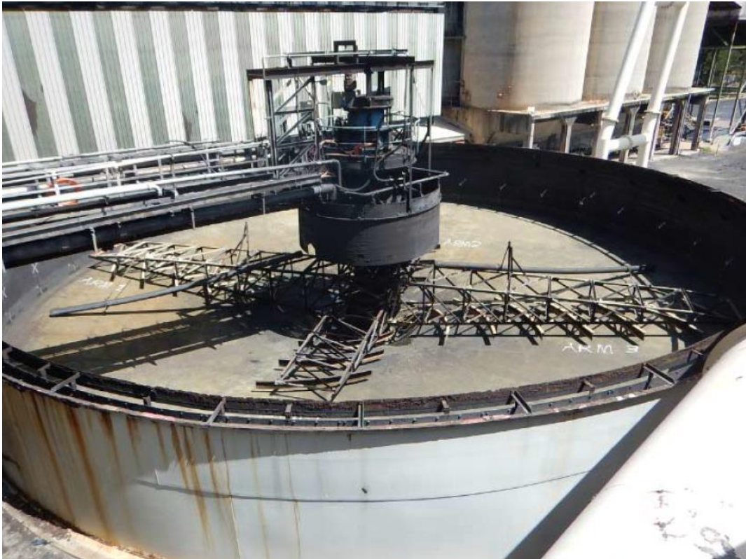
Figure 1: Existing WCCPP coal product thickener before upgrade (emptied)
