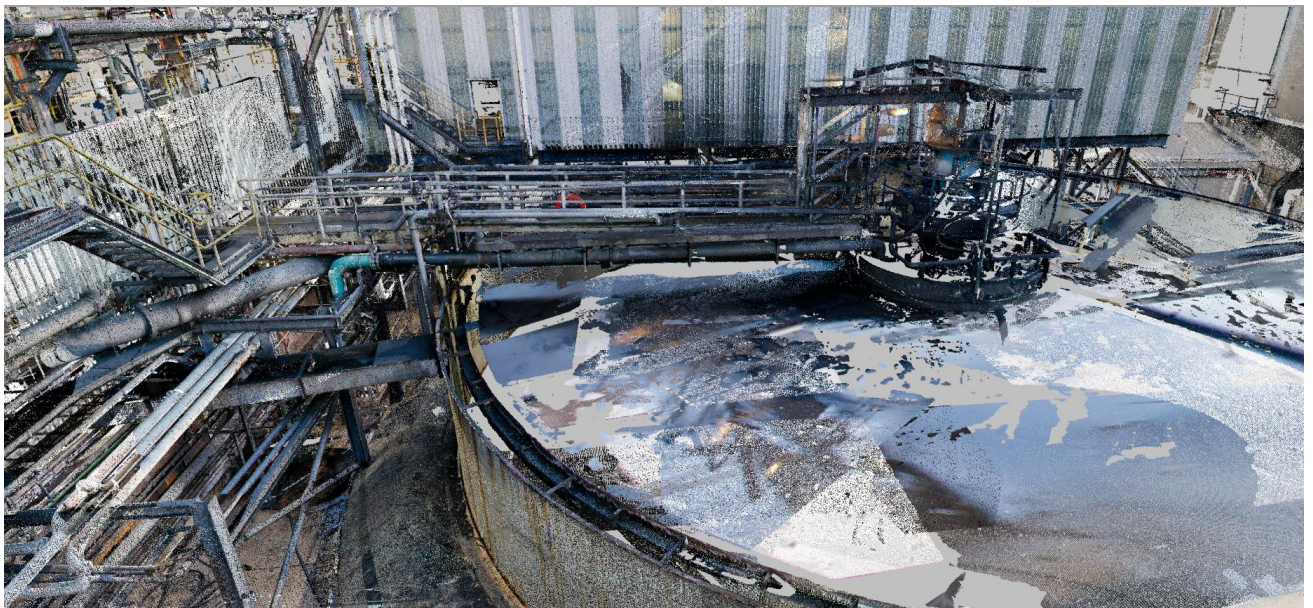
Figure 7: View generated from 3D laser scan data showing pre-upgrade thickener with half-length bridge
