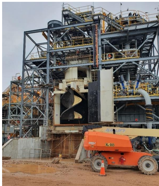
Figure 9 - VTM-4500-C circuit during construction
