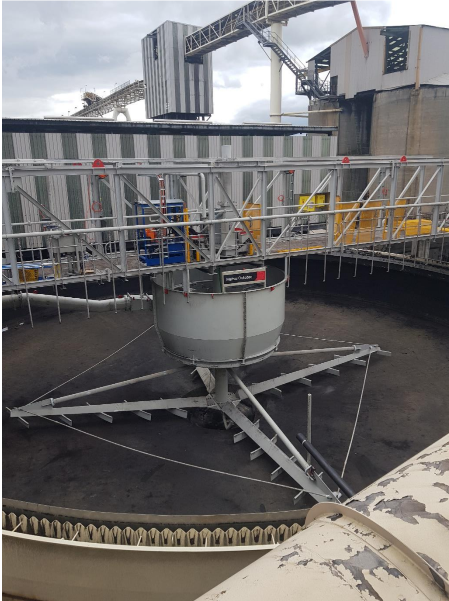
Figure 12: Coal Product Thickener at completion of installation.
